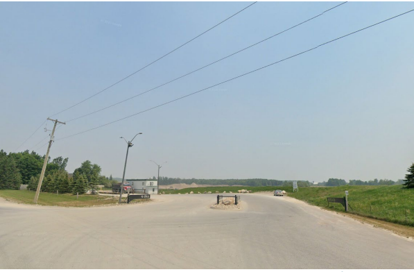
Existing southern entrance from 4 th Line
