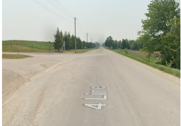
4 th Line at the North Driveway, Looking South
