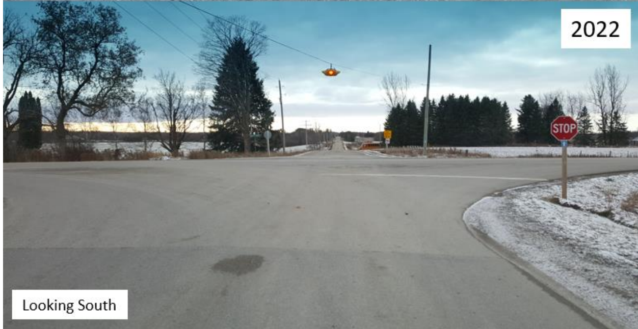
Exhibit 22: Stop Bar Along 4th Line at Dufferin Road 17
